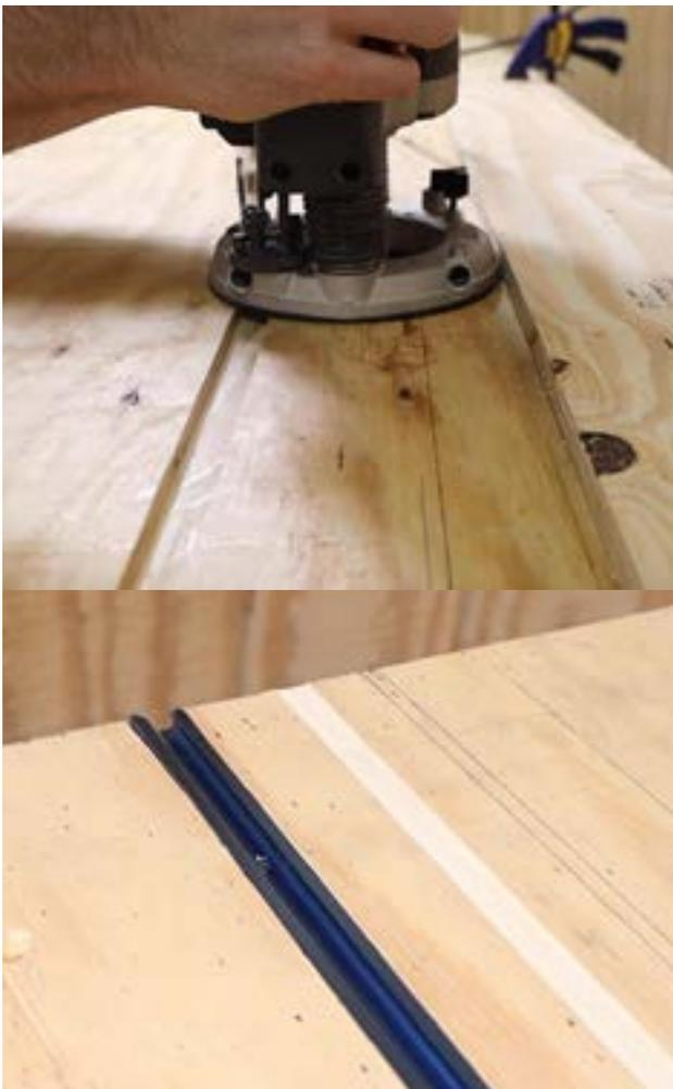
**Step 10:** Set the router depth to about 1/16", and run another groove about 2" behind the T-Track. This groove will be used to install the measuring tape that the Stop Block uses.
